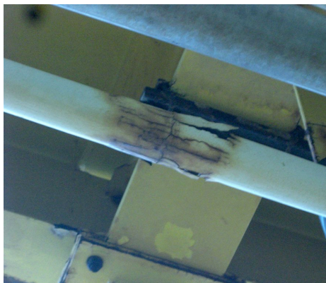
Figure 1: Original Visual Inspection
